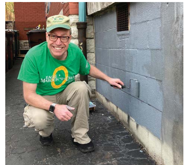
Paul Wesselmann – graffiti remediation
