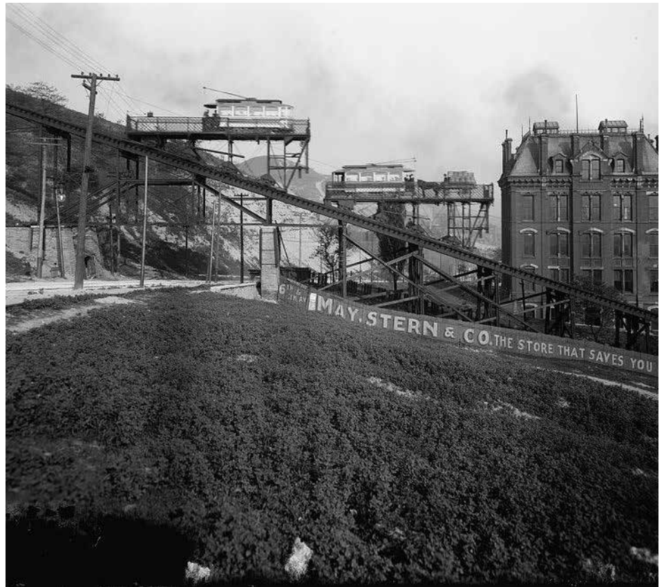
“Bellview Incline” crossing above Clifton Ave. passing the old Medical College, supported by stone pillars still visible today.
