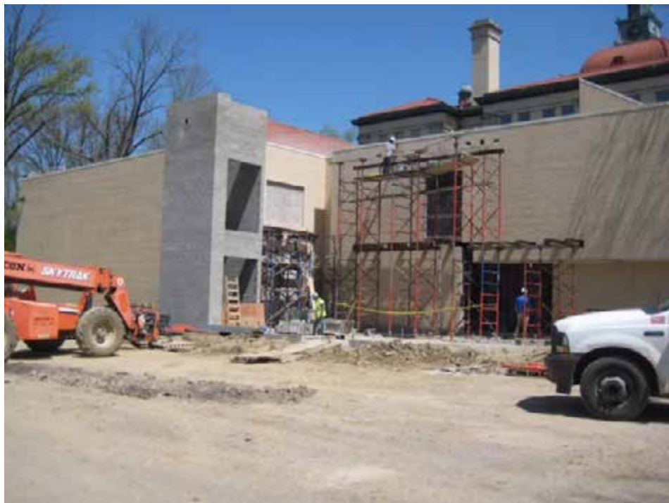
Front of Clifton Recreation Center under construction
