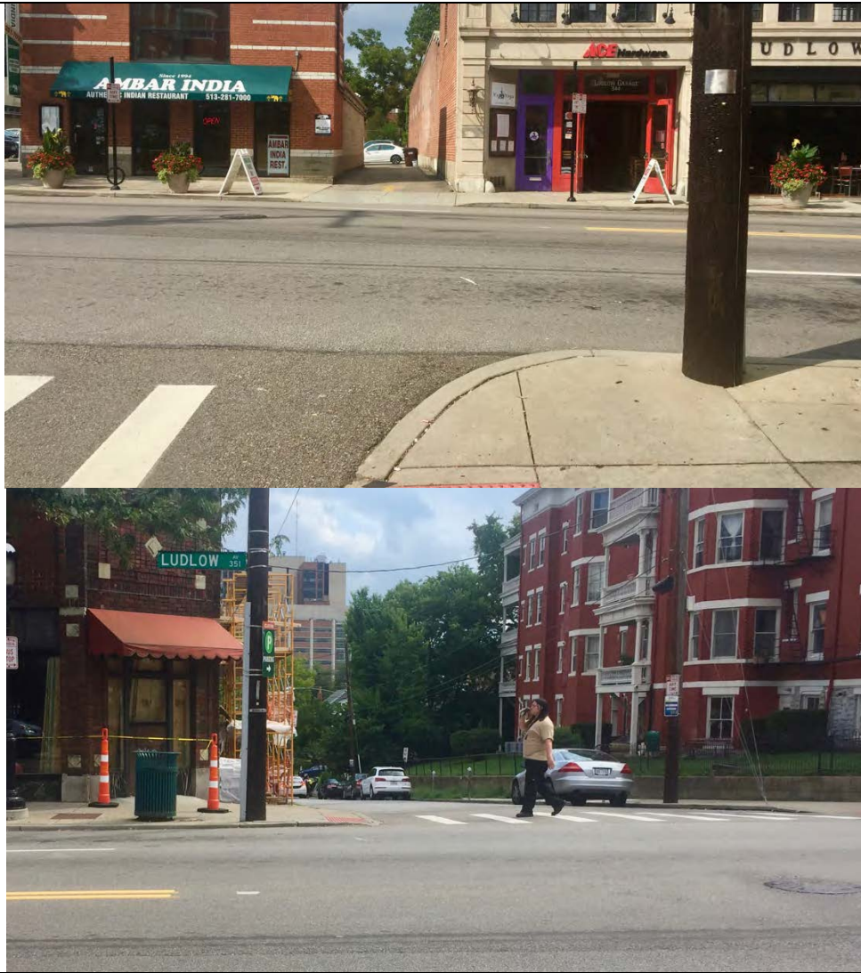
Figure 9 Street-level views of Ludlow Ave at Ormond Ave
